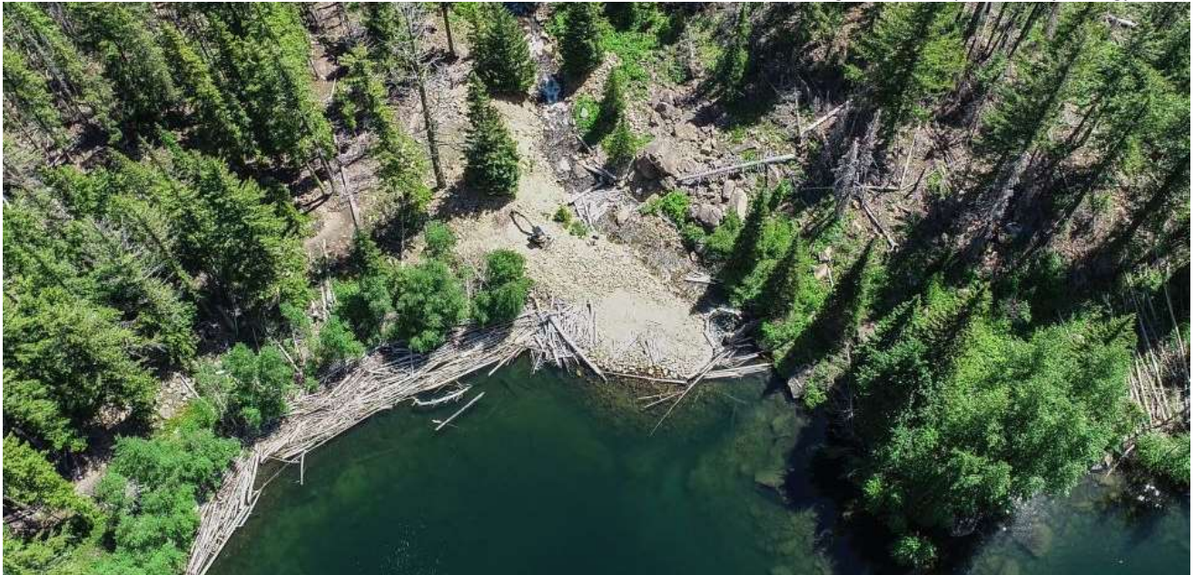
Figure 9-2. Eightmile Lake Dam after 2018 emergency repairs
