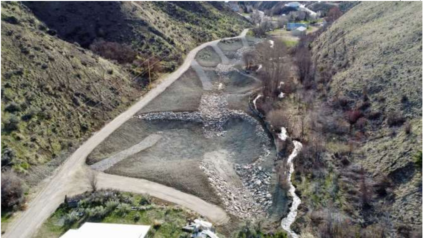
Figure 12-1. Number 1 Canyon Debris Basin
